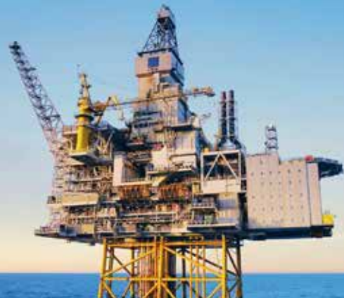
Oil & Gas Pipe Line
